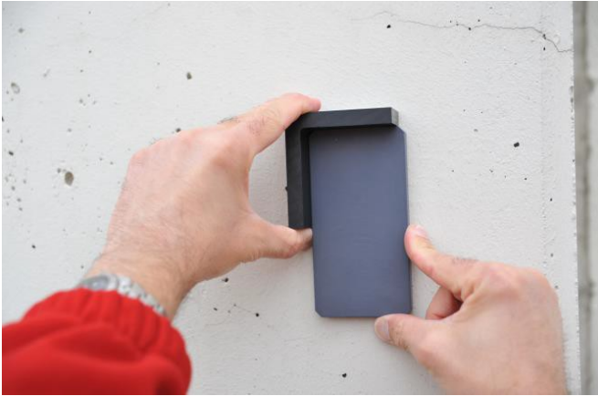
Figure 12: 3/8" Spacer with L Shaped Template
