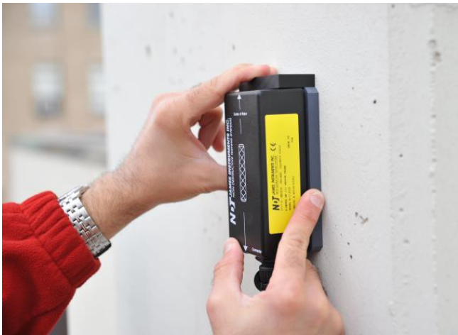
Figure 13: Locating Rebar with Spacer
